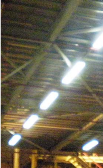
High frequency fluorescent lighting
